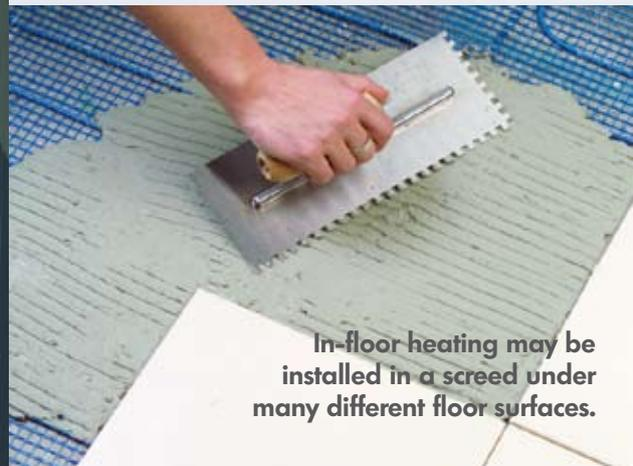
**In-floor heating may be installed in a screed under many different floor surfaces.**
