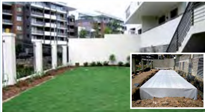
Holroyd Apartments, Sydney
