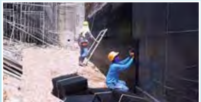
Retaining Wall, Singapore
