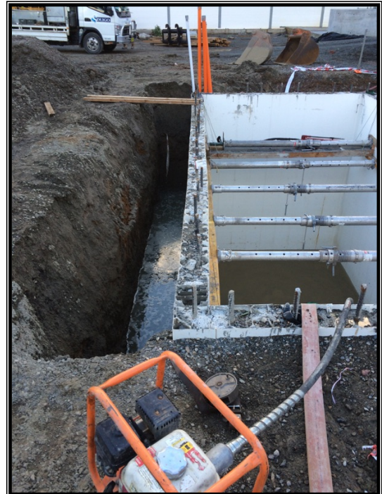
Photo No: 2 – Shows Rectified Wall
