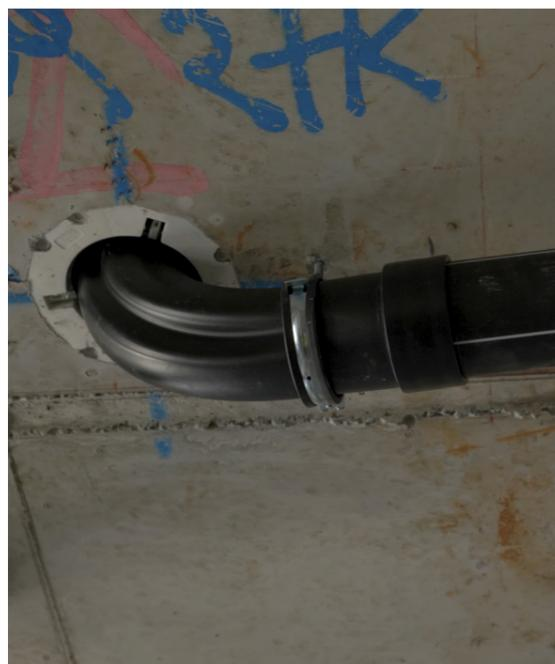
Geberit BottomTurn bend supports the horizontal pipelines without slopes for up to 6m, creating loftier ceiling heights.
