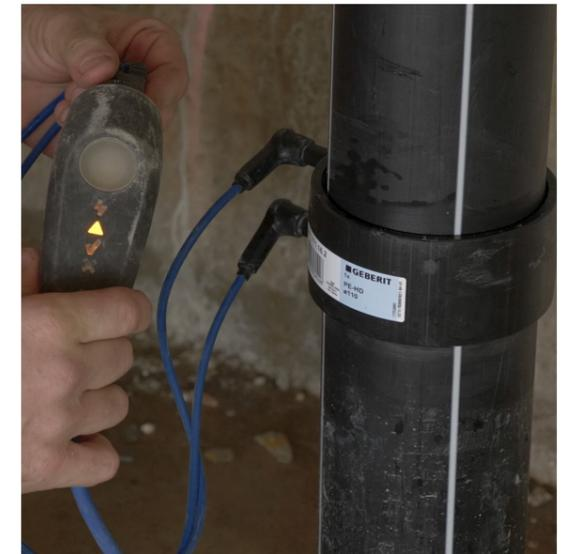
Only one electrofusion joint per stack using Geberit ESG3 machine makes it safe and easy to use.
