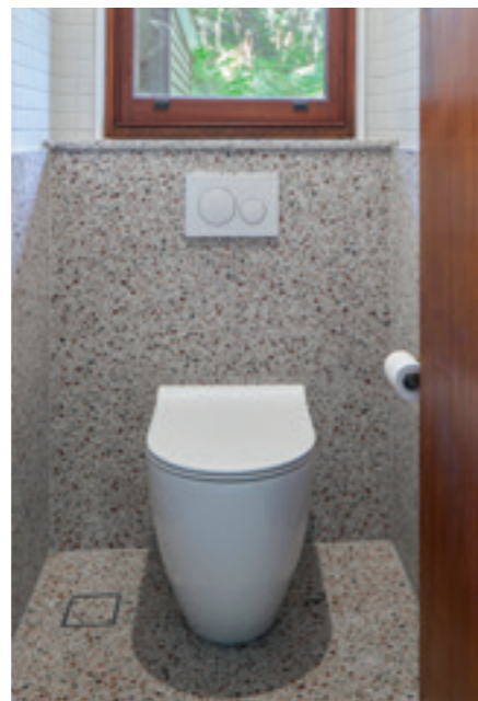
← Geberit Kappa Con- cealed Cistern with Sigma20 White Matt Tone-in-Tone Flush Buttons.
