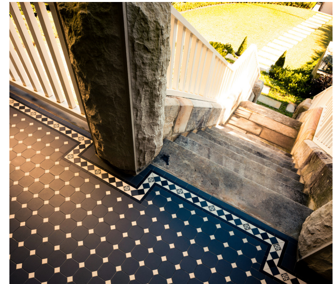
Detail of a front verandah of a house in Sydney's affluent suburb of Mosman. TTF's tessellated octagon and dot pattern in black and white, with border trimmings that include TTF's 'Bordeaux Neative' tessellated encaustic.
